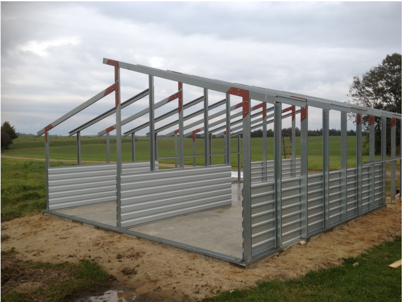
Figure 1. Here is the metallic frame capable of withstanding earthquakes of large magnitude or typhoon magnitude 5. It is sitting on a cement base that can be pre-fabricated. Future users can be trained rapidly to install and build this future house they will inhabit for a period of time.
