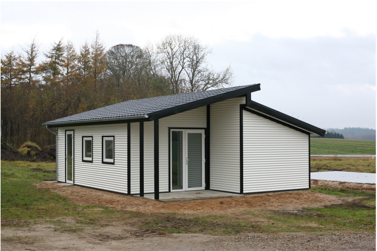
Figure 2. The external panels can be installed in any climate and would not be attacked by termites. In very warm climates we can use other types of panels that will reflect more than 40% of the heat generated by sunshine.
