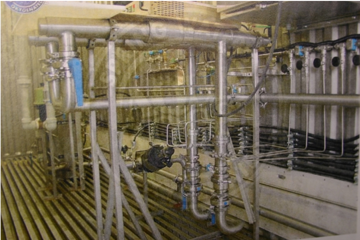
Figure 5. The above illustrations, shows the machines we use to decontaminate and/or to oxygenate the water, It can generate 136 liters per minute . This unit is used as a mobile unit that delivers oxygenation or decontamination where needed. You can deliver oxygenated water to an hospital or to a farming unit or to a place where you need to decontaminate the water. This mobile unit can contain up to 10 units of water treatment. One unit generates approximately 6,000,000 liters per month.
